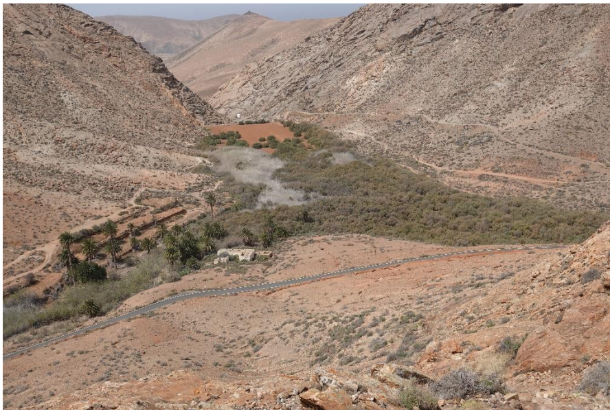
The dam. Over time, due to the loss of rain water, the dam has silted up.
